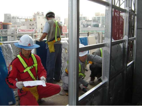
Steel Curtain Wall
